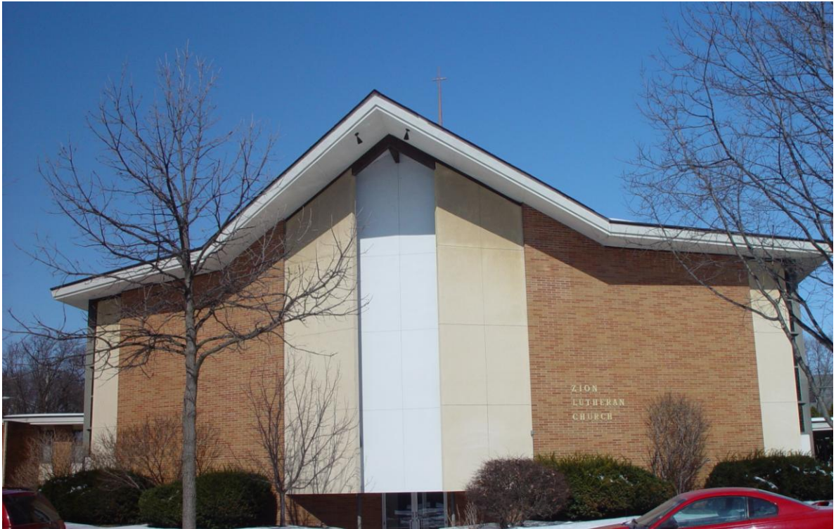
View from the South - 2010
